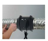
Attach the ducts with clamps.
