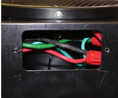
Figure 14: Wire connections carefully pushed into wiring compartment.
