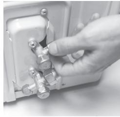
**STEP 3** Locate and remove the protective threaded caps on the "in" and "out" refrigerant ports on the outdoor unit.
