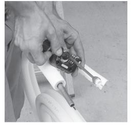
**STEP 2** Once the proper length for the line set is determined, leaving enough room for the final connections, use the copper line cutting tool to remove the factory flair and fitting, so that the copper line set ends are bare. Remove any burrs as needed. Repeat this step for all copper lines to be attached to the outdoor unit.
