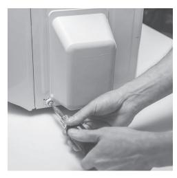
**STEP 1** On the outdoor unit of your mini-split, locate and remove the plastic refrigerant line cover. This is usually attached to the unit with one or more Phillips-head screws. Put cover and screws aside until self-installation is complete.
