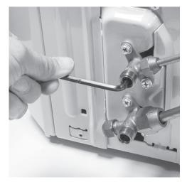
**STEP 14** Locate and remove the refrigerant valve caps on the outdoor unit and set aside. Using a 5mm hex key, open the valves to release the refrigerant into the line set(s).
