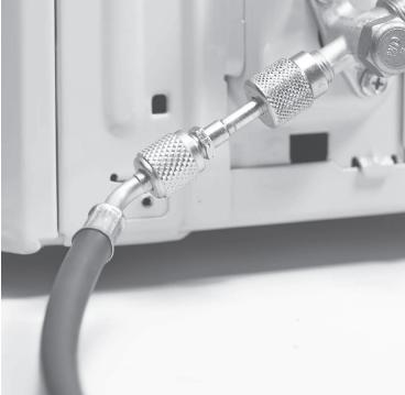
**STEP 11** On the mini-split outdoor unit, remove and set aside the protective cap on the refrigerant port. Thread on the other end of the hi-pressure tubing to hand tight to the refrigerant port.
