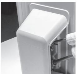
**STEP 15** Remove the vacuum line and replace all the caps on the outdoor unit, tightening with the crescent wrench or channel lock pliers. Be sure to replace the plastic refrigerant line cover and screws.
