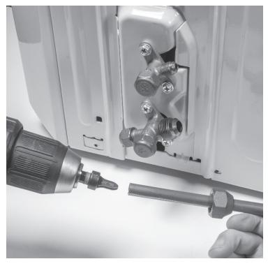
**STEP 4** Slip the fitting onto the cut copper line and using the appropriate size flaring bit with a power drill, flare the end of each copper line.
