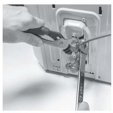
**STEP 5** Gently insert the flared end of the copper refrigerant lines into the sockets, making sure the line is fully seated in the socket, using 2 wrenches to tighten the fittings.
