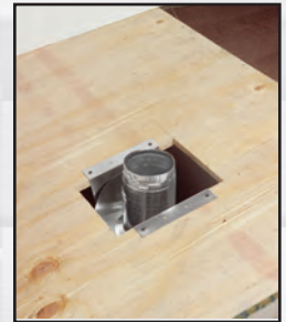
Push pipe through vent support.
