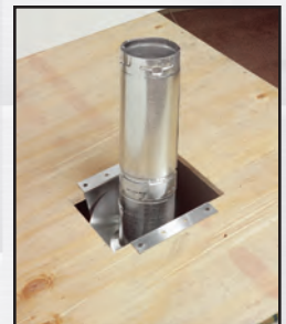
Continue adding pipe sections – supports up to 90 lbs.
